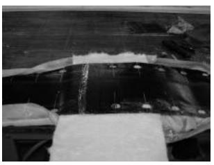
Figure 12 – Position insulation covered plywood board.
