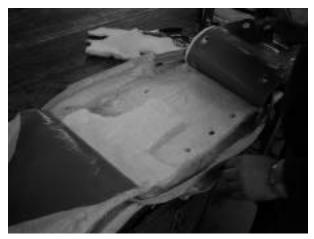
Figure 4 – Overlapping Insulation Layers
