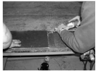
Figure 20 – Grind taper into elastomer ply.
