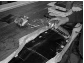
Figure 15 – Fold cuffing over edges and secure with glue
