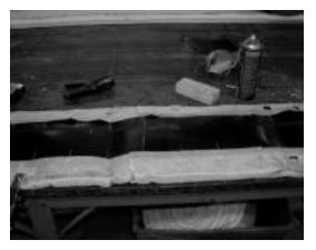
Figure 17 – Completed splice of flexible element.
